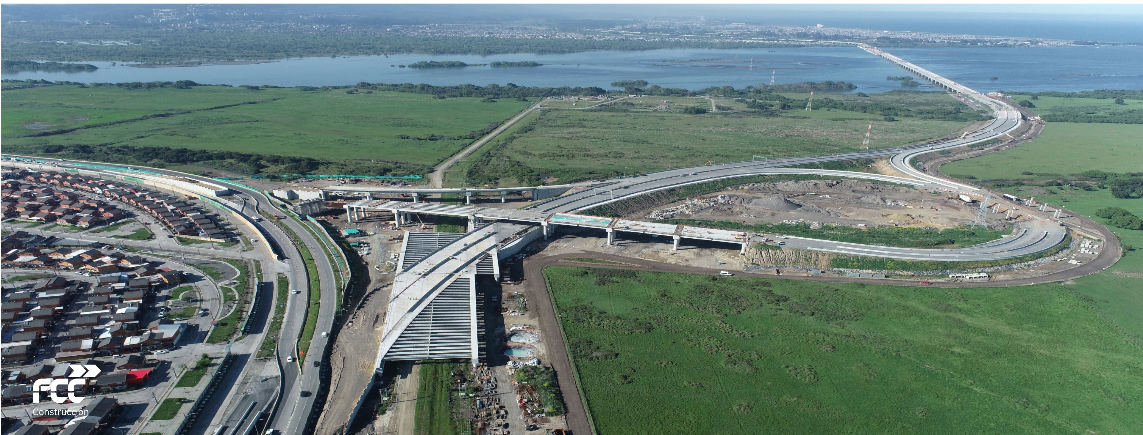
Ponte Industrial, Chile
